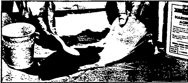
Fig. 58—Applying Resin Mixture to Fiberglass
